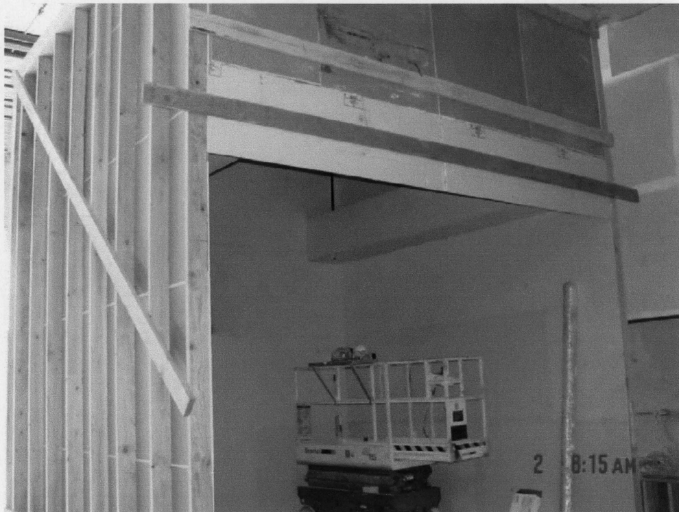
Photo 6: Front View of Room with Soffits Installed.
