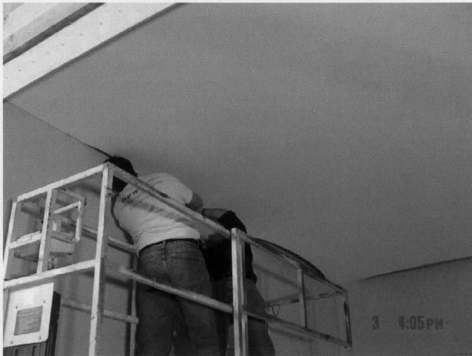
Photo 8: Installation of Stretch Ceiling Material.
