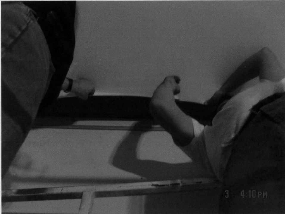
Photo 9: Installation of Stretch Ceiling Material.
