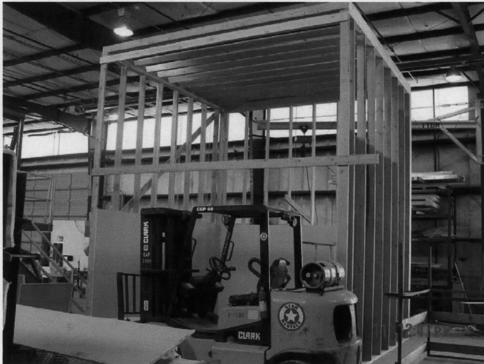
Photo 2: Another Construction Photo of Room.
