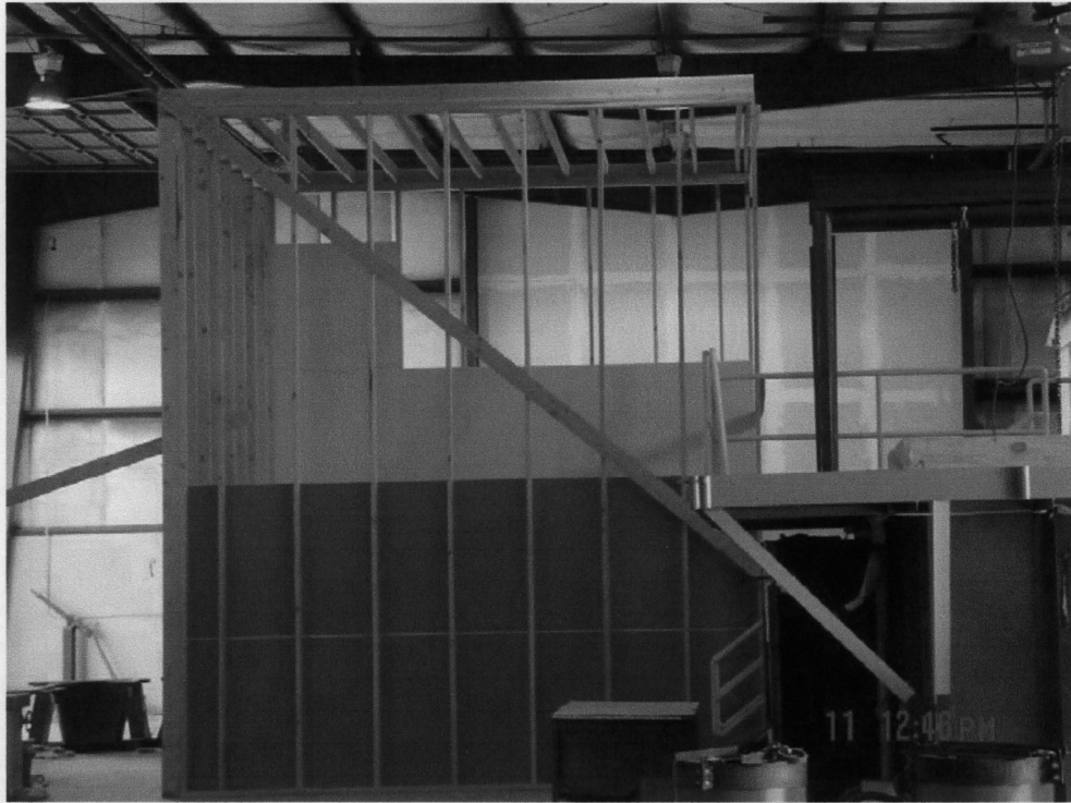
Photo 1: Room Being Constructed.
