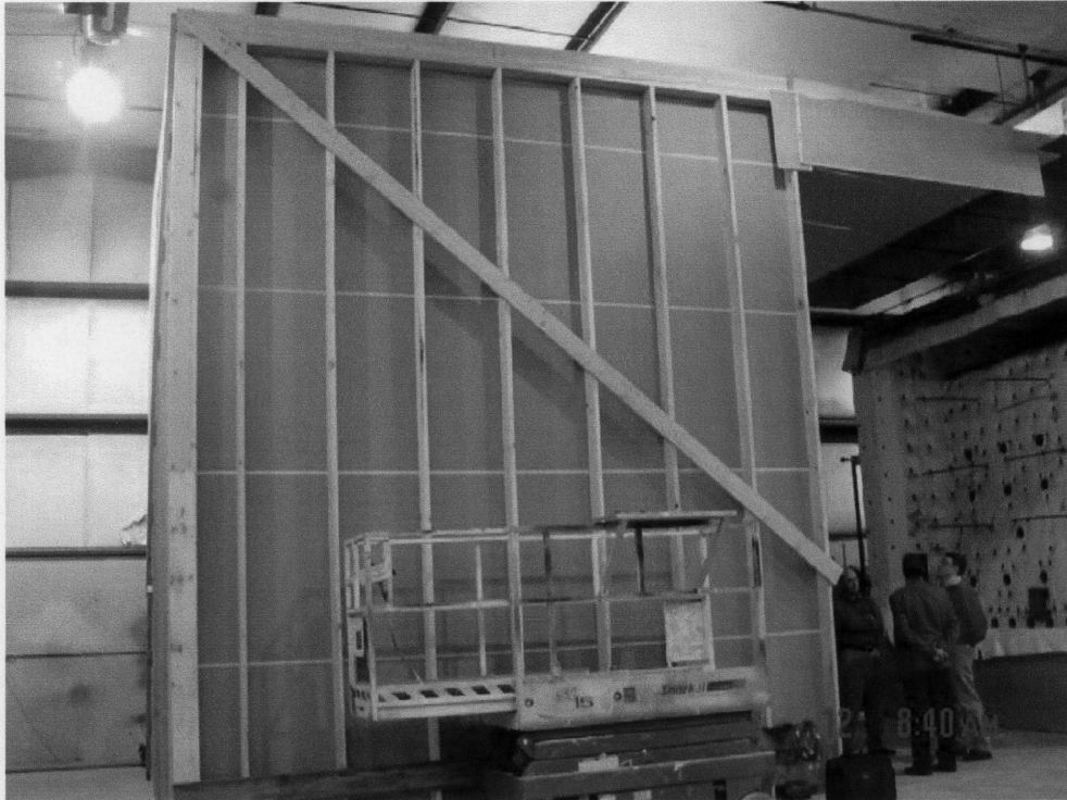
Photo 3: Room Construction Complete.
